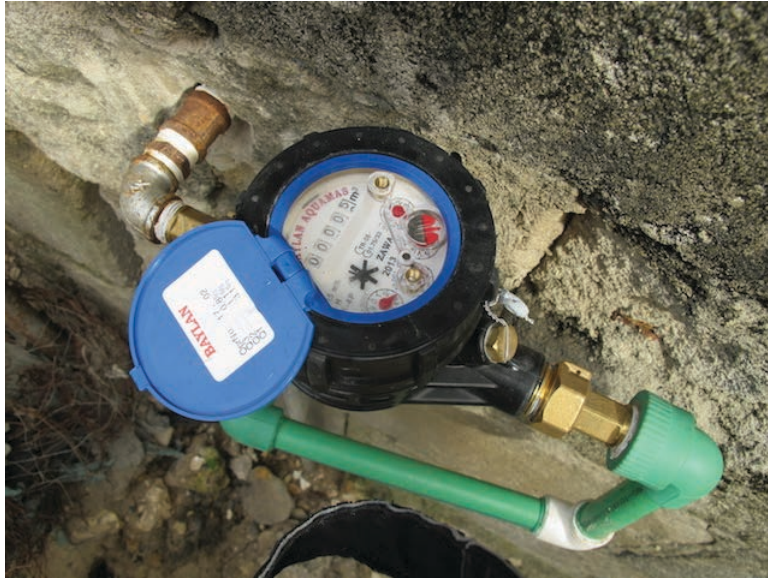
Picture: Customer meter installed for each household in Zanzibar
